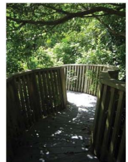
Example shows path connection that can connect between two topographically steep areas
