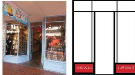
Recessed entrances with glazing atop a solid stall board make a special feature of the entry point and create interest on the street.
