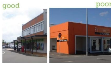
The verandahs of the BNZ building (left) are good as they extend the width of the footpath and are supported by posts. Although a modern interpretation, the BNZ example also shows a parapet line and extended vertical structural features at the corners. The building entrance is emphasised with a change in verandah height. The example on the right is poor as it has no verandah and has no parapet features.
