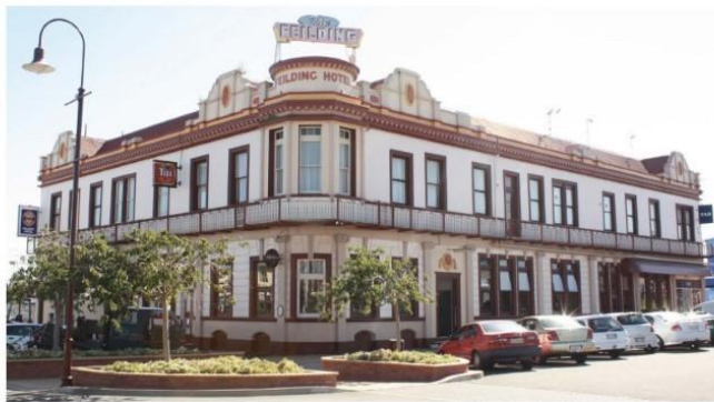
Feilding Hotel, 9 Manchester Square (constructed 1875-1910)
