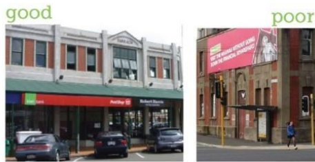
The above example (left) is good because the signs clearly identify the building and businesses within it, but are discreet and do not extend to the area above the verandah or interrupt the facade details. The example above (right) is poor as the sign is not advertising products available on site and it obscures building facade features.
