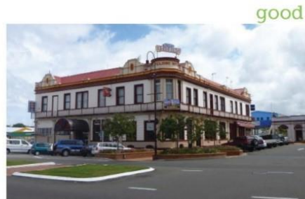
The facade of the Feilding Hotel is a good example as its openings are placed symmetrically, and as a corner building it has doors to both frontages
