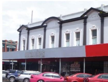
The good example above shows modulation created by a series of structural bays - highlighted in the dark colour in this instance. The bay 'modules' continue up the building to the top.
