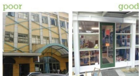
The two examples of external strengthening above contrast. The poor example (left) has cross braces (painted green) that run diagonally counter to the building's modulation. The good example (right) has a portal type bracing that fits with the door and window frame proportions and is painted the same principal white colour to de-emphasise it.
