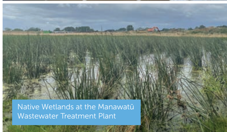
Native Wetlands at the Manawatū Wastewater Treatment Plant
