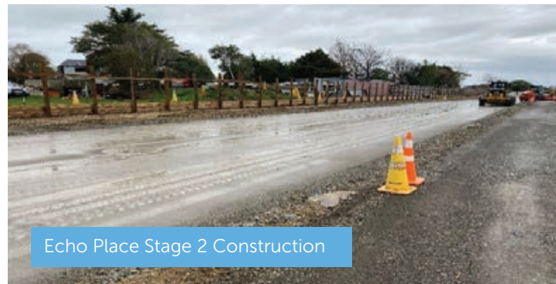
Echo Place Stage 2 Construction
