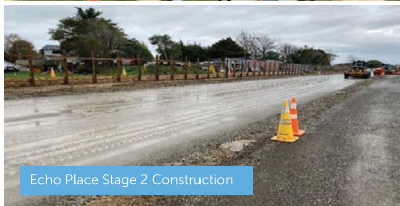
Echo Place Stage 2 Construction
